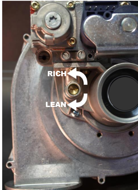
Illustration 2 - Air/Gas Mixture Ratio Screw
